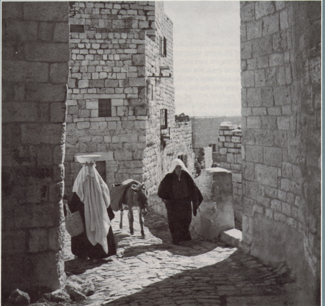
The New Testament Church
